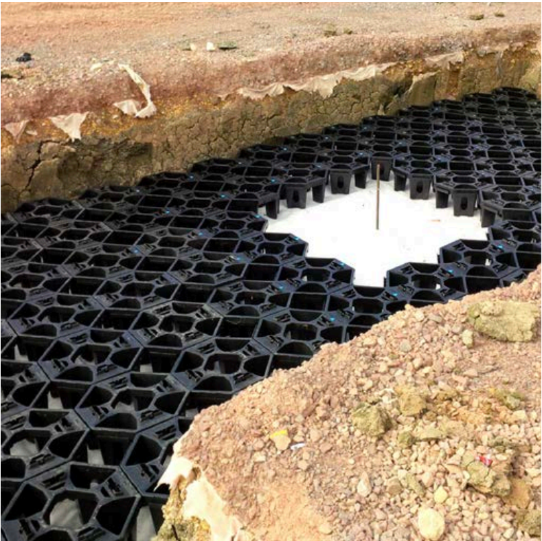
Example of stormwater management tree rooting cells
